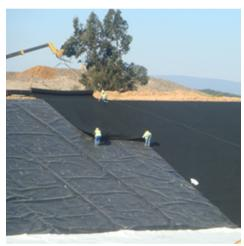
Geosynthetics are materials used in civil engineering, in which at least one of its components is made from a synthetic or natural polymer, in the form of a sheet, a strip or a three-dimensional structure, used in contact with soil and/or other materials in geotechnical and civil engineering applications. They have replaced traditional materials, significantly increasing the safety factor, improving the performance of works and reducing construction and maintenance costs.
